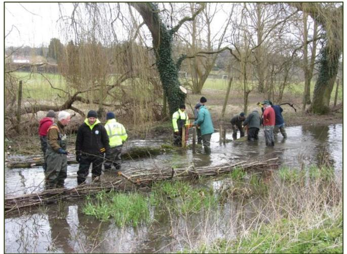
**From this: Narrowing an over-wide silted channel using large woody debris and brush.**
