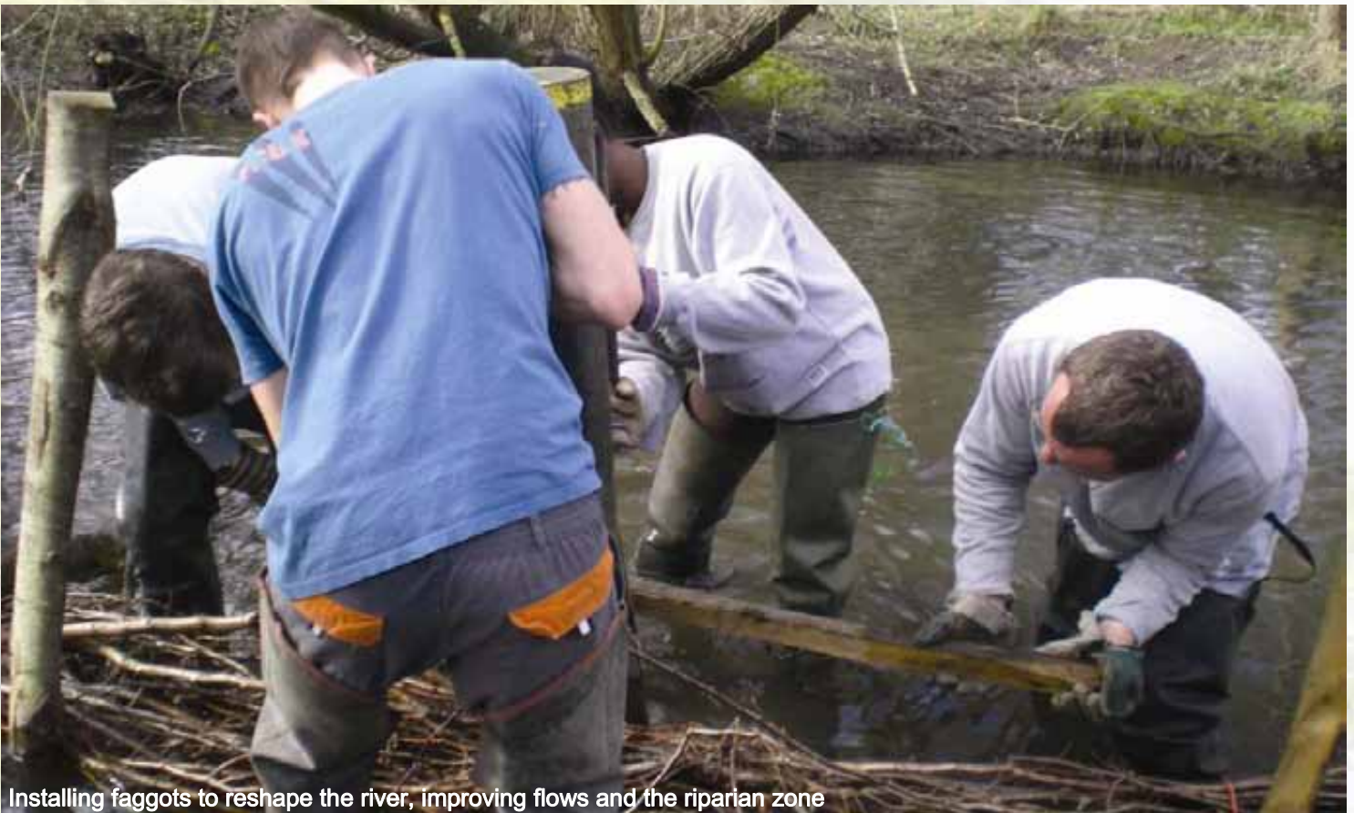
Flow deflectors, such as these, help restore flows on overly straightened sections of river
