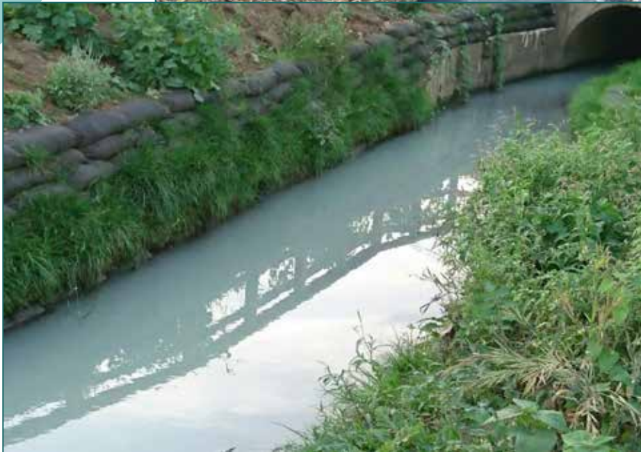
Trunk sewers overflowing into new river restoration project 29.09.16
