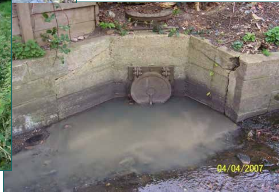
Sewage effluent overflowing from a dual manhole and entering the surface water sewer before draining into the river
