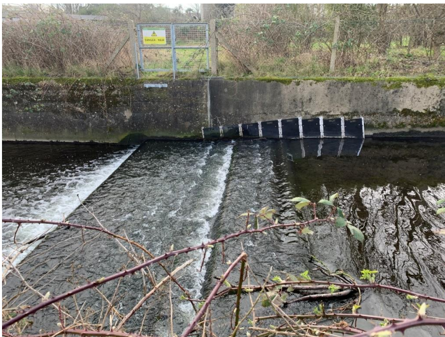
Figure 4.1: Image of improvements made to Mereway Barrier 1.
