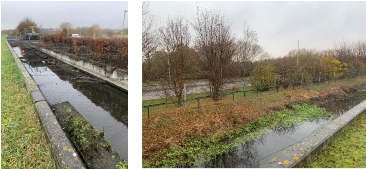
Figure 6.3: (Left) Image of gabions and large woody material installed in the Upper Duke of Northumberland's River by Heathrow Conservation and Biodiversity Team. (Right) Image showing the growth of marginal vegetation planted in the Upper Duke of Northumberland's River at Heathrow.
