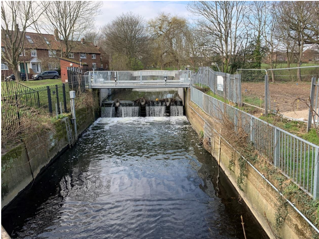
Figure 4.2: Image of Mereway Barrier 4 taken prior to improvement works commencing (10/03/2022).
