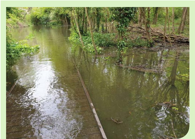
Figure 2.2: Flooded boardwalk in Donkey Woods. Deliberately designed localised flooding in parks allows space for water during heavy storms and reduces the risk of property flooding.
