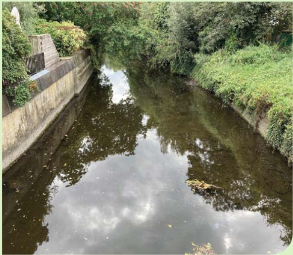
Figure 4.1a: Straightened, over-wide, over-deep and reinforced channel with no natural geomorphological function and little habitat to support wildlife.
