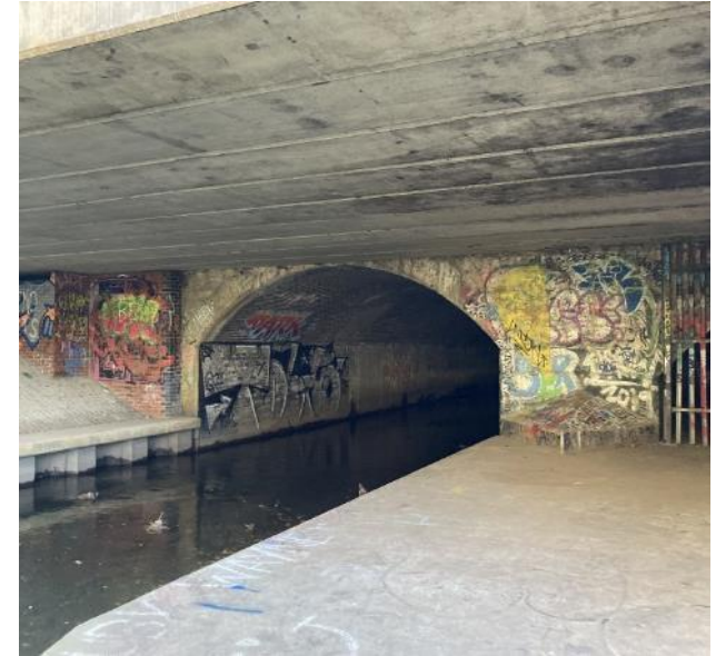
The Crane flows through a railway underpass at Feltham Marshalling Yards
