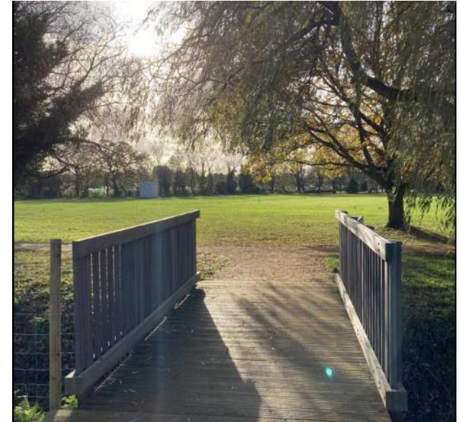
A bridge over the Yeading Brook in Headstone Manor
