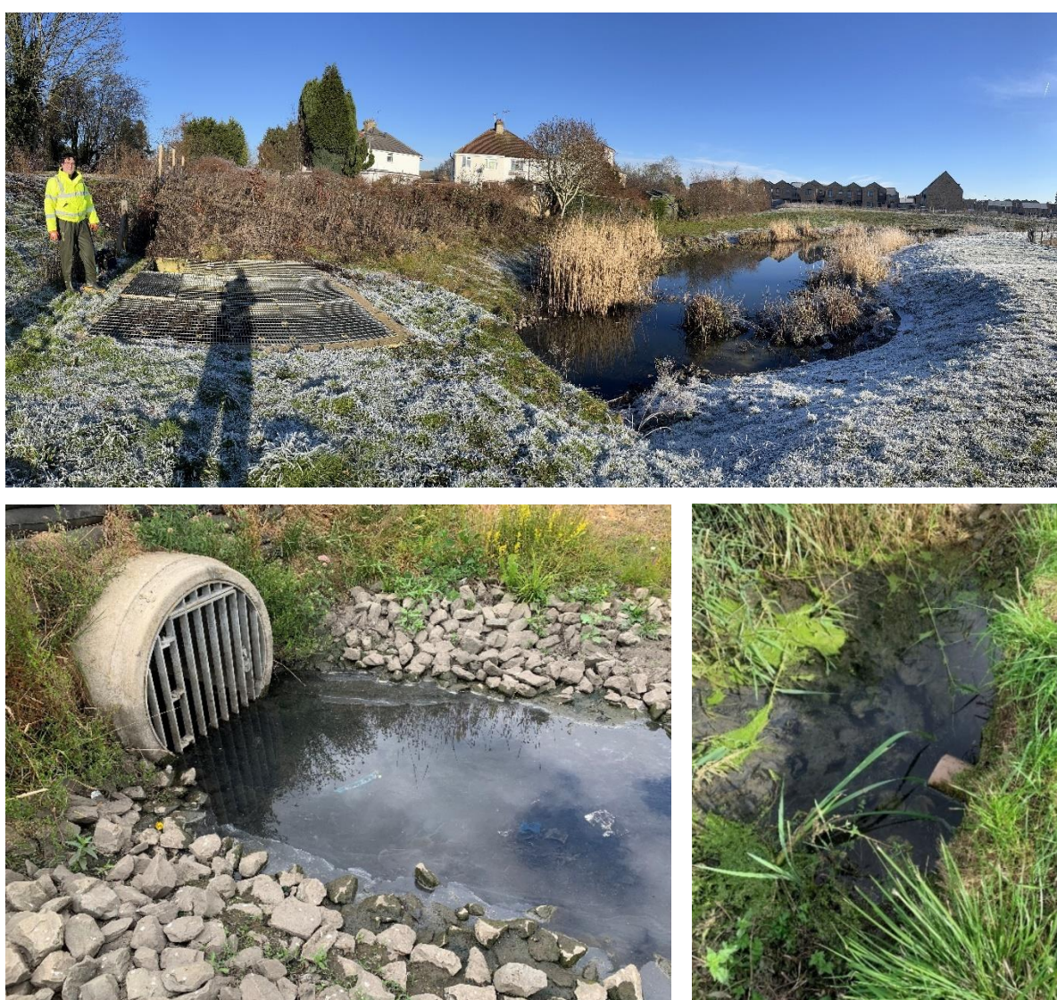
Figure 2.1: (Top) Wetland inlet, with inlet sondes installed below metal grating. Credit: Adrian Butler, Imperial College London (Bottom left) Location of the wetland inlet spot samples. (Bottom right) Location of the wetland outlet sonde and spot samples.
