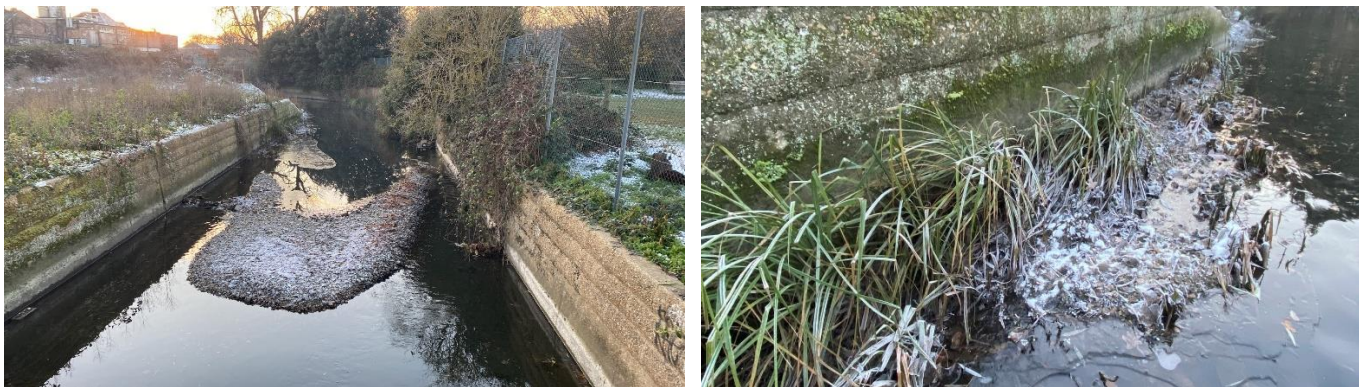
Figure 4.4: (Left) Bar created by gravels that have been washed out of the restoration site due to heavy rainfall and subsequent high flows. (Right) Gravels retained within the planted areas of the restoration site. Credit: ©Wild Future
