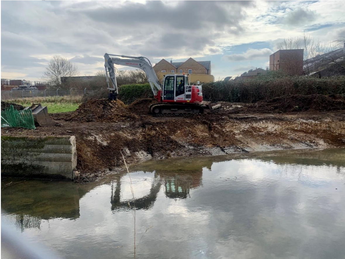
Figure 4.1: Digger removing soil and material to create the backwater.
