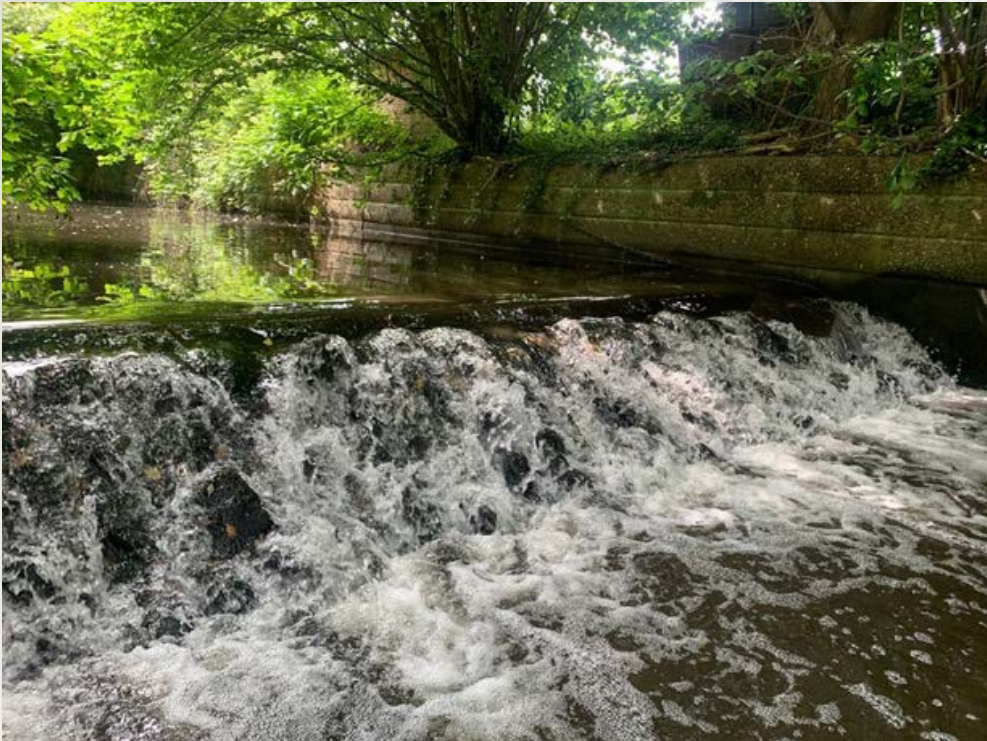
Weir at the downstream end of Moormead Recreation Ground
