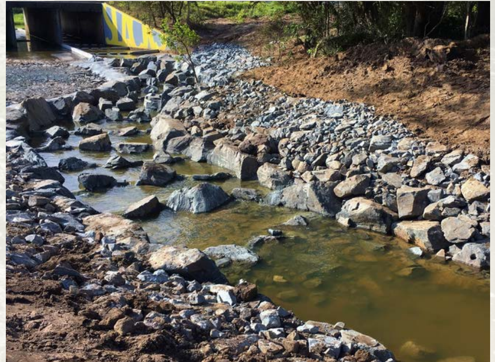
Example of a rock ramp fish pass
