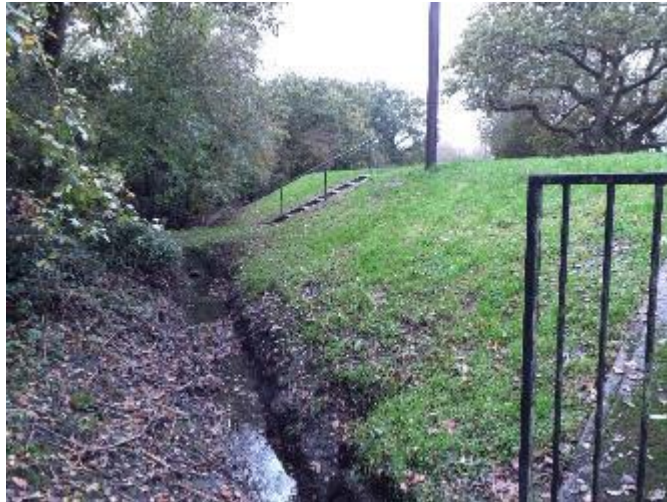
Figure 4.47 Flood embankment delineating Charville Lane FSA. Note the tributary in the foreground; this occupies a relict meander of the channel.
