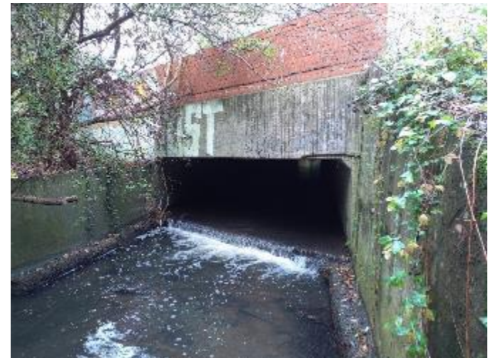
Figure 4.12 Step weir at the lower limit of Reach 1. The bed and banks of the Brook are reinforced with concrete as it flows beneath the A437.
