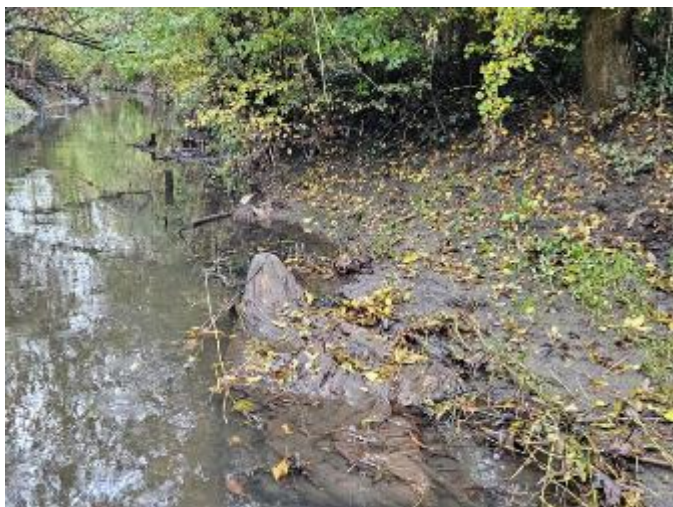
Figure 4.16 Evidence of former restoration attempts; berms built along the channel have failed leaving wooden stakes used to secure brushwood fascines.
