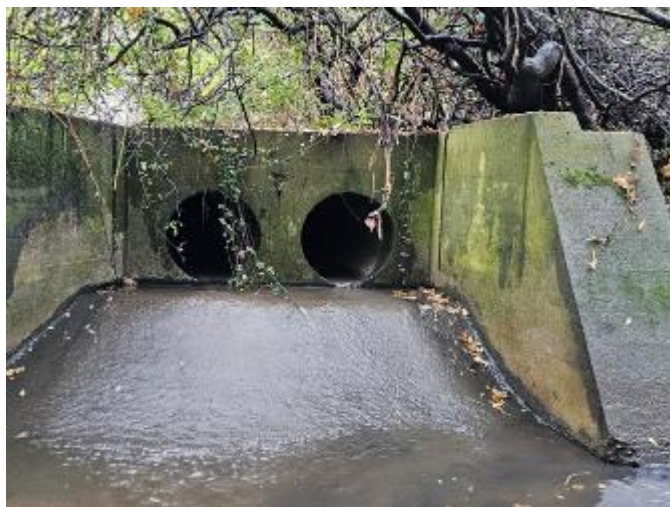
Figure 4.17 A culverted tributary flows into the channel in the upper reach. This likely conveys runoff from roads and residential properties south of the Brook.
