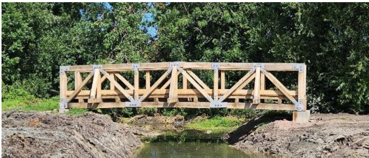
Figure 5.9 Example of a hardwood bridge being installed over a realigned channel. Source: cbec eco-engineering UK Ltd.
