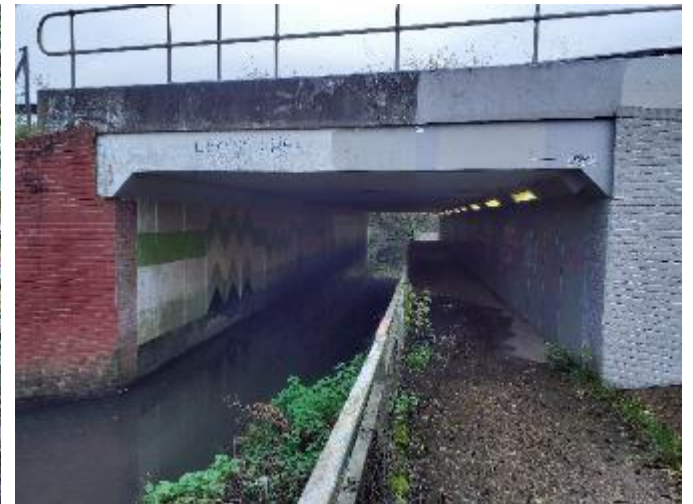
Figure 4.9 Looking downstream along the channel at the A40 road bridge. The beds and bank of the channel are reinforced with concrete.
