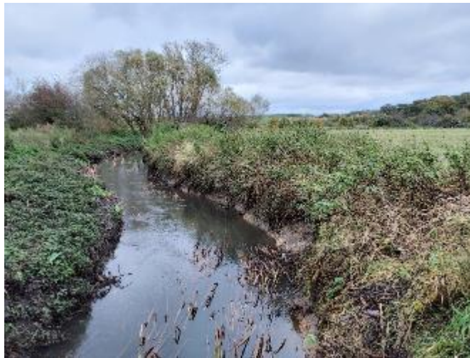
Figure 4.34 Sections of the channel exhibit erosion (either toe-scour or shear face)
