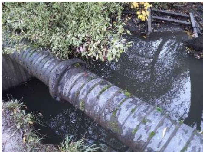
Figure 4.30 Raised pipe just downstream of the gauging station. This is a mains distribution pipe owned by Affinity Water.
