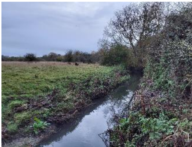
Figure 4.4 ↑ Upstream extent of Reach 1. The channel has been extensively modified; it has been straightened, resectioned, and is now disconnected from its floodplain. Marginal and in-channel vegetation is largely absent or poorly developed.
