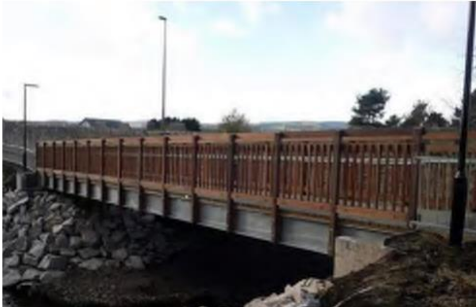
Figure 5.10 Example of a steel and timber bridge suitable for vehicles that could be installed (Photo courtesy CTS Bridges).
