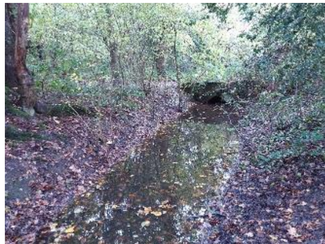
Figure 4.24 Drainage ditch running parallel to the channel through the TRB floodplain. This is set back ~30 – 40 m from the bank top.
