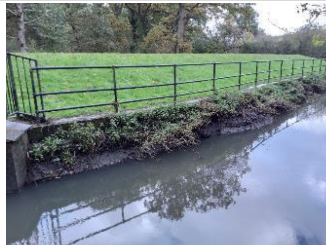
Figure 4.59 Flood embankment bordering the TLB of the channel downstream of Charville Lane FSA.
