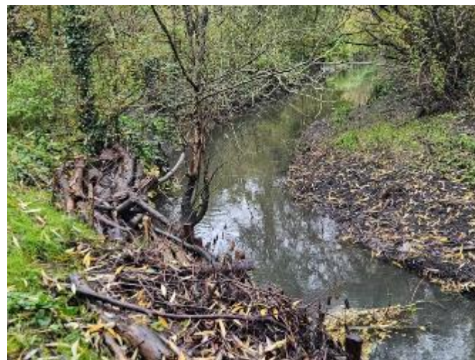
Figure 4.18 The channel exhibits toe scour (minor to moderate in severity). Short sections of erosion protection measures consisting of logs/brush have been installed.
