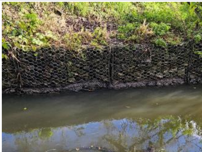
Figure 4.58 Rock filled gabions line both banks of the channel immediately downstream of Charville Lane FSA.
