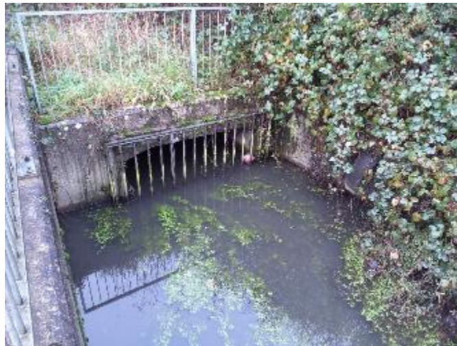
Figure 4.8 A culverted tributary flowing into the channel immediately upstream of the A40 road bridge. Note the trash guard.
