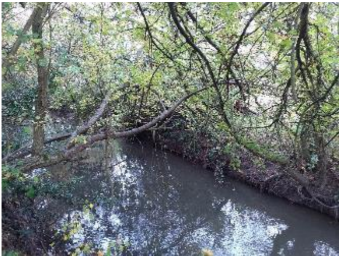
Figure 4.7 Trees form a dense hedge along the channel. Note the limited understorey and bare earth of the banks. Erosion (toe scour) is also evident.
