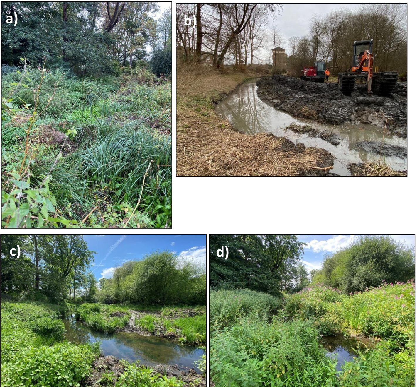
Figure 3 , De-silting and de-shading carried out on Crane Park Island to improve the site for water vole, a) prior to work commencing, b) improvement work being carried out winter 2022/23, c) spring 2023 and d) summer 2023. Photo credit – Steve Marshall
